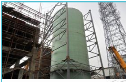
Flue Gas Desulfurization Tower
